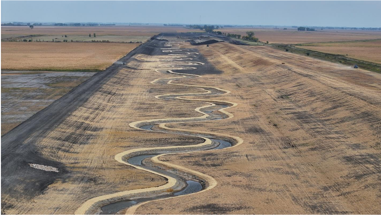
Photo Caption: The BdSWD's Mustinka River Restoration Project, September 2023. Excavated soils provide material to construct embankments for flood storage in the 19,000 acre-foot Redpath Impoundment. (Photo Credit: Moore Engineering).
